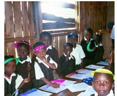
The old sawmill building classrooms are not favorable to learning
