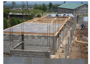
The new classroom building is going up fast
