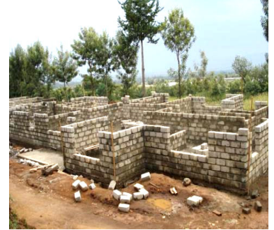
One of the two new children's homes now under construction
