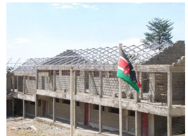
Twenty new classrooms under construction
