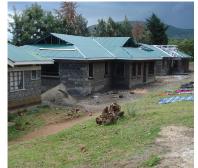
The two new children's homes under construction
